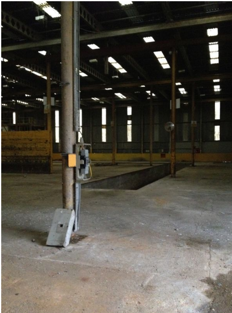
Photo 4.1: DS Smith site, interior of building
