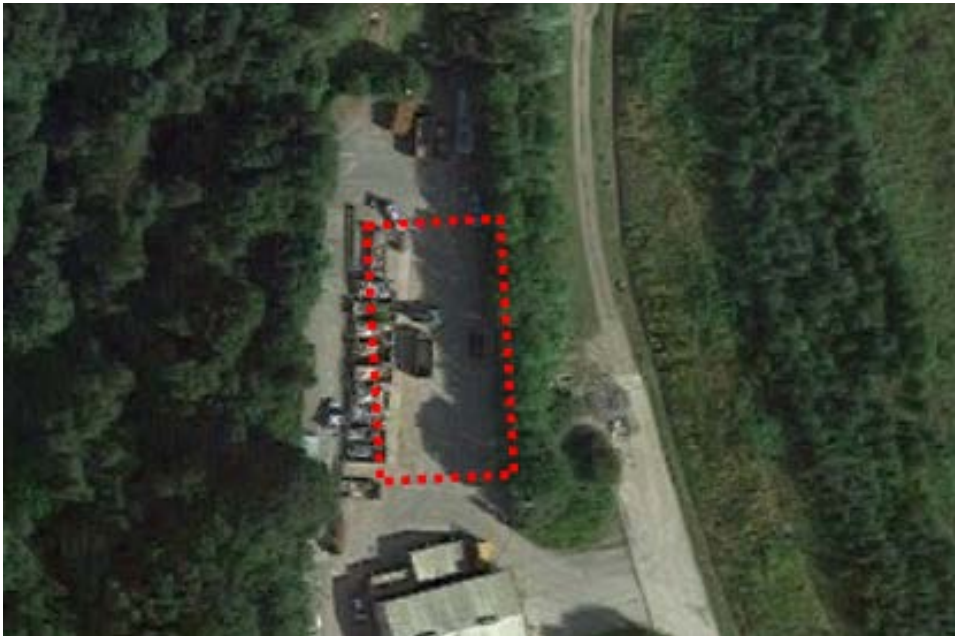
Trehir Phase 2 Works
