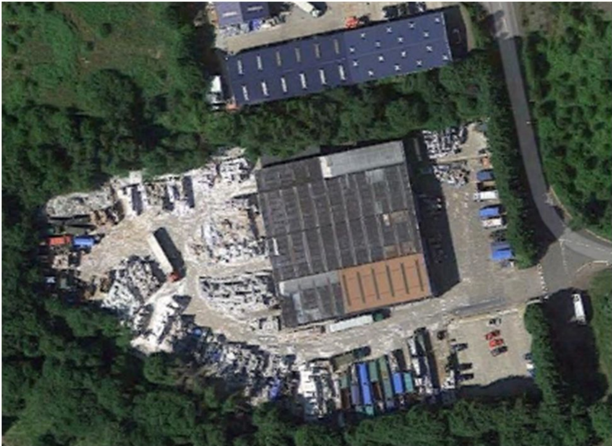
Note: this photo was taken when the site was being used to bulk and process paper
